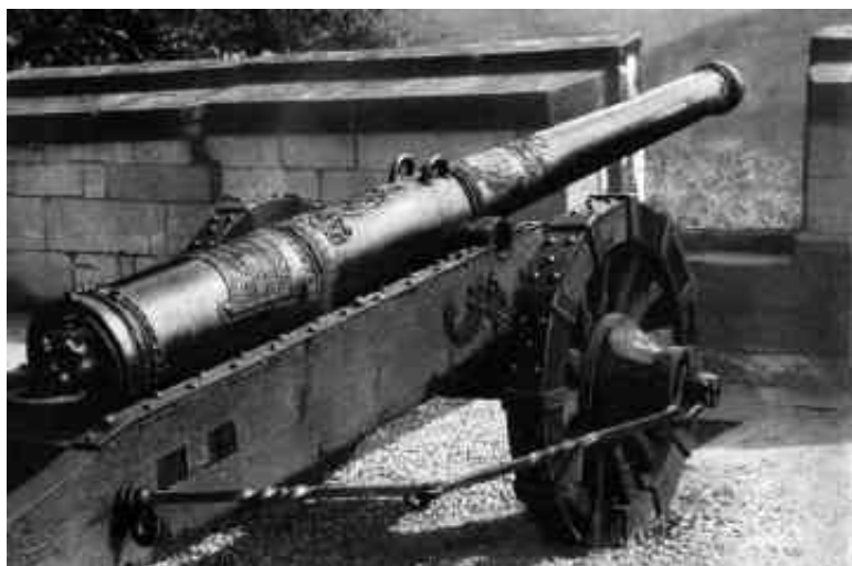
FIG. 8: SCHÖNE TREIBERIN, A SAXON FIELD GUN (FELDSCHLANGE) FROM 1521. SIX-POUNDER, CALIBRE 90 MM. NOTE THE TRUNNION IN THE MIDDLE OF THE BARREL UNDER A SEMICIRCULAR IRON PLATE
